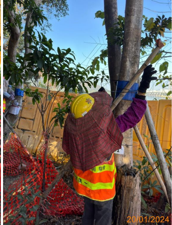
18: Re-adjustment of staking
