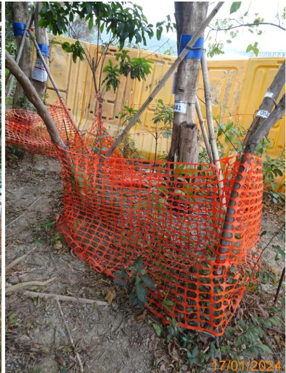
20: Temporary protective fencing for U041, U042 and U043e
